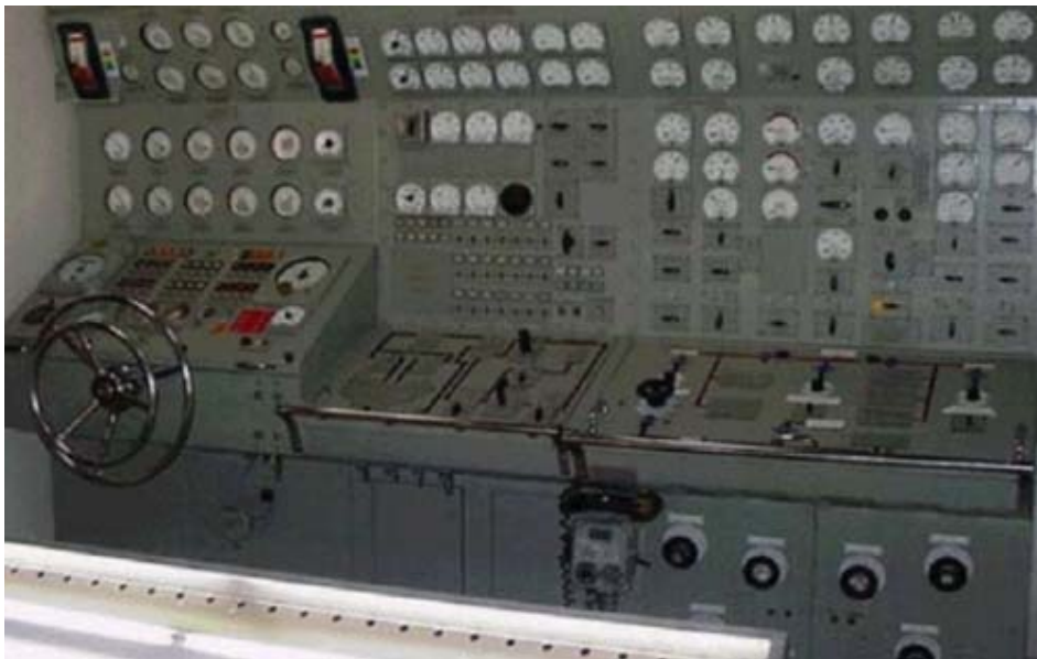
TYPICAL MANEUVERING ROOM CONTROL PANELS STEAM PLANT (SPCP) - REACTOR PLANT (RPCP) - ELECTRIC PLANT (EPCP)
